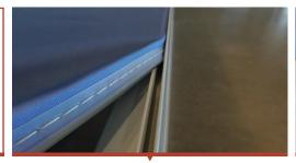
**8.** Attach the fabric by pushing the silicone edges in the grooves.
