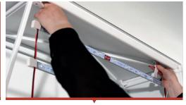
1. Hold the LED curtains against the frame with the 2. Attach the LED curtains to the frame by mark 'UP' towards the topside.
